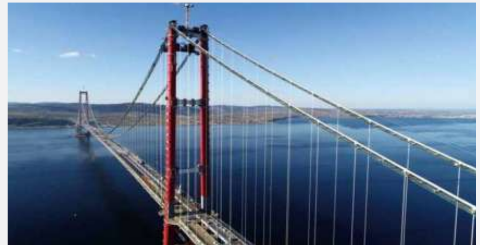
1915 Çanakkale Bridge Construction Blasting and Coating
