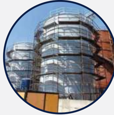
SCAFFOLDING INSTALLATION IN ALL AREAS
