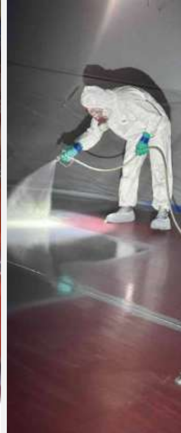
APPLICATION OF FINISHING COAT PAINT
