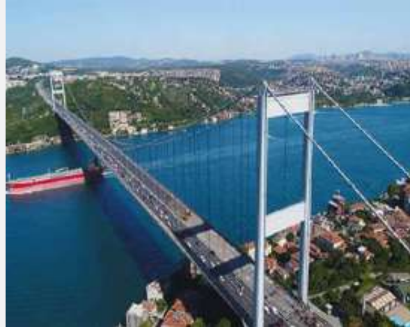
15 Temmuz Şehitler Bridge Deck Abrasive Blasting and Membrane Installation
